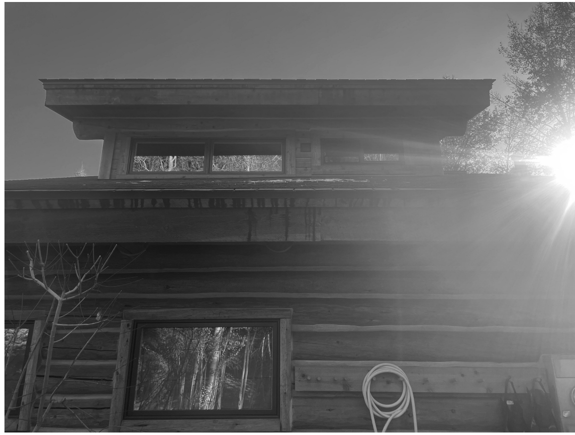
PHOTO #3 - NEW ADDITION ROOF TO ATTACHE AT UPPER RIGHT OF PHOTO
