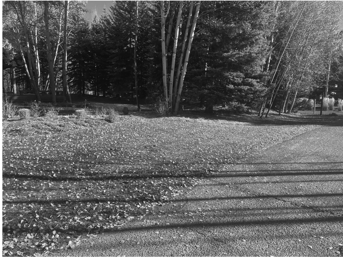
PHOTO #9 - AREA OF WIDENED ROADWAY TO CREATE REQ. FIRE DEPT. PULL OUT AND ACCESS TO FIRE HYDRANT
