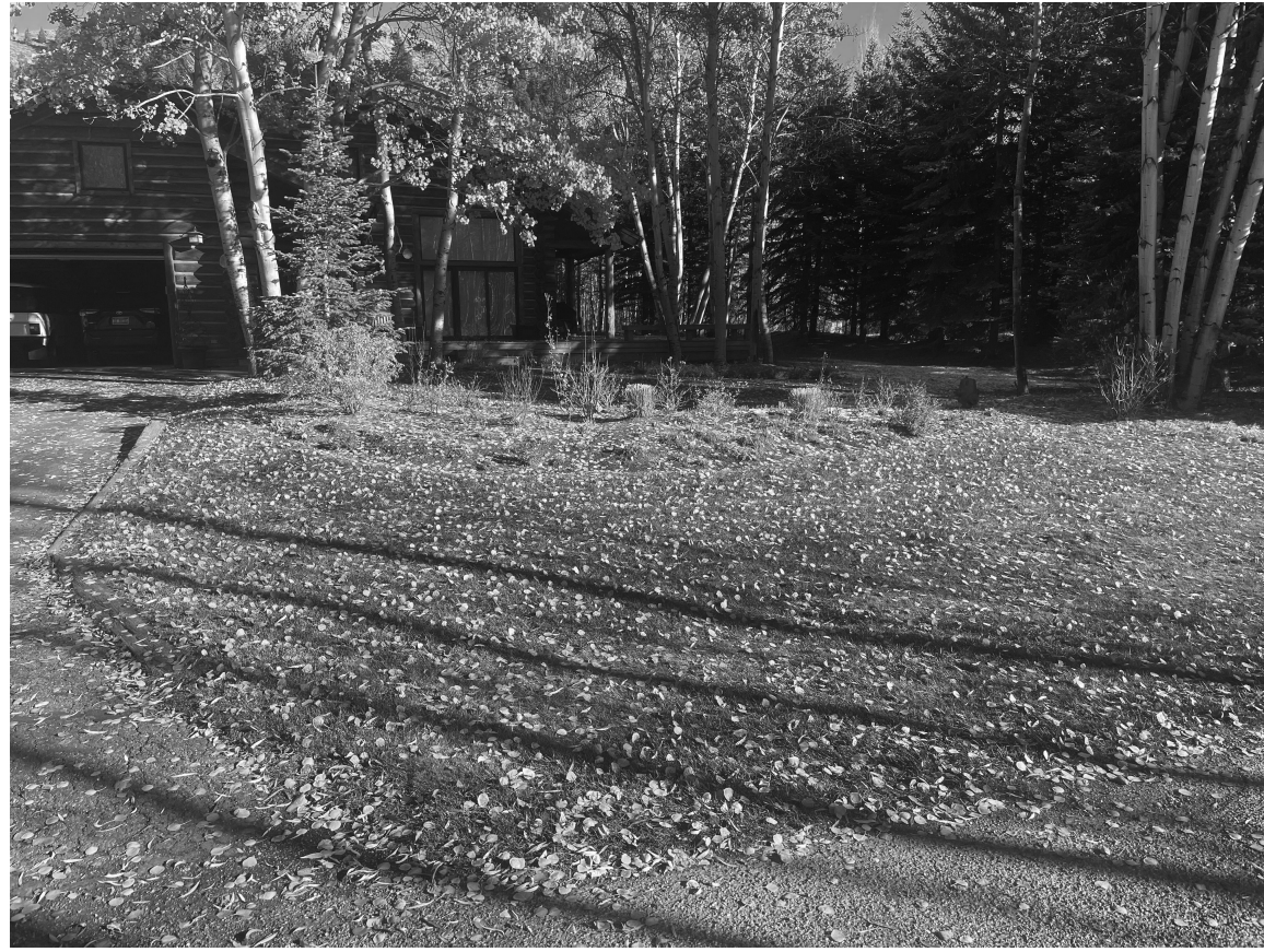
PHOTO #10 - AREA OF WIDENED ROADWAY TO CREATE REQ. FIRE DEPT. PULL OUT AND ACCESS TO FIRE HYDRANT
