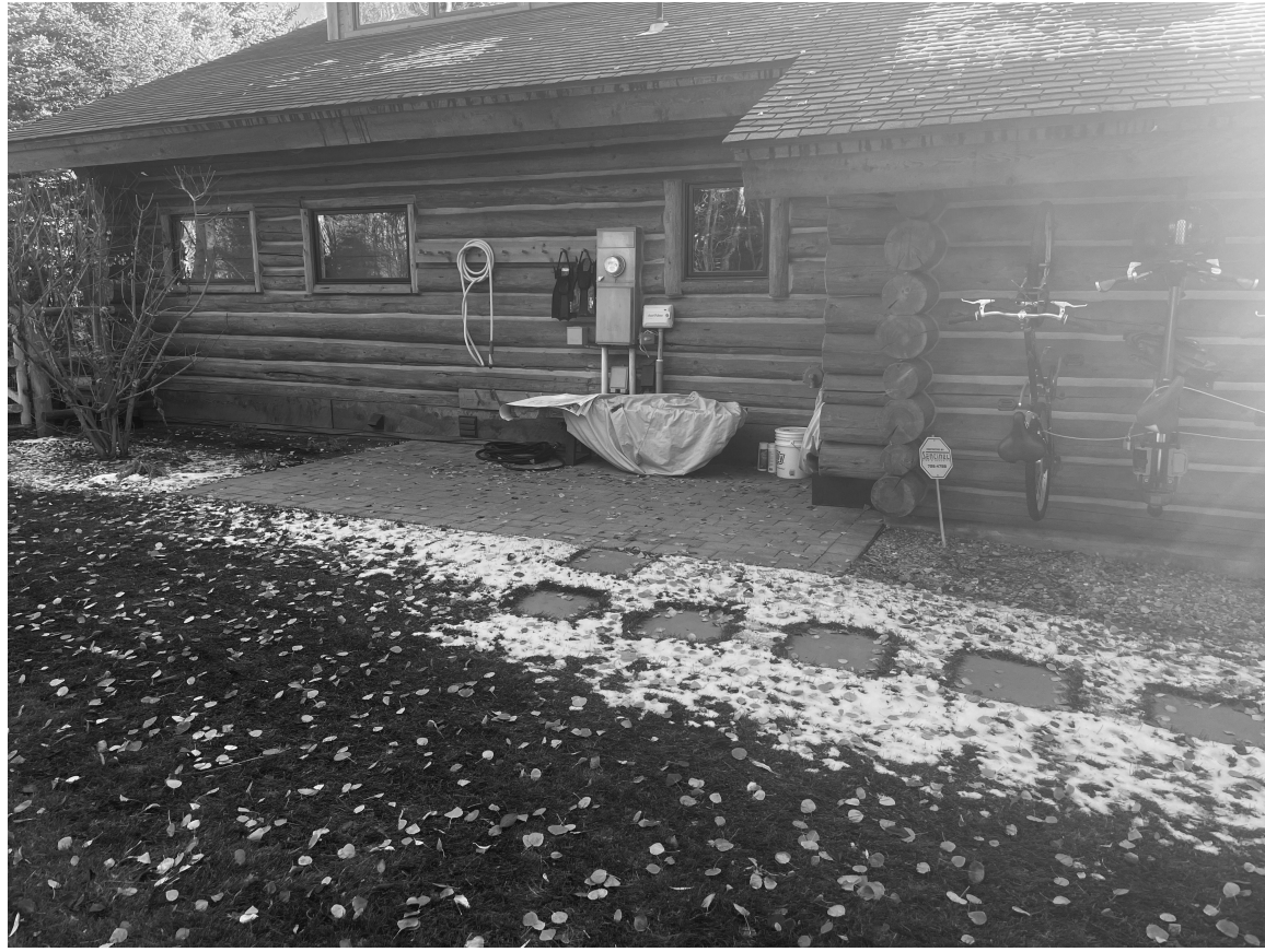
PHOTO #7 - AREA OF ADDITION
