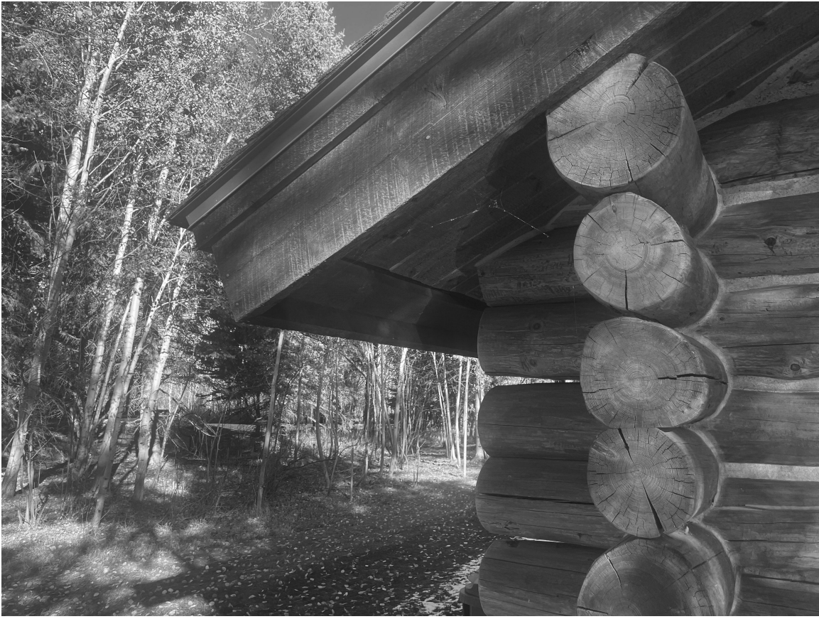
PHOTO #6 - ADDITION TUCKS IN STARTING IN/BEHIND THIS LOG CORNER
