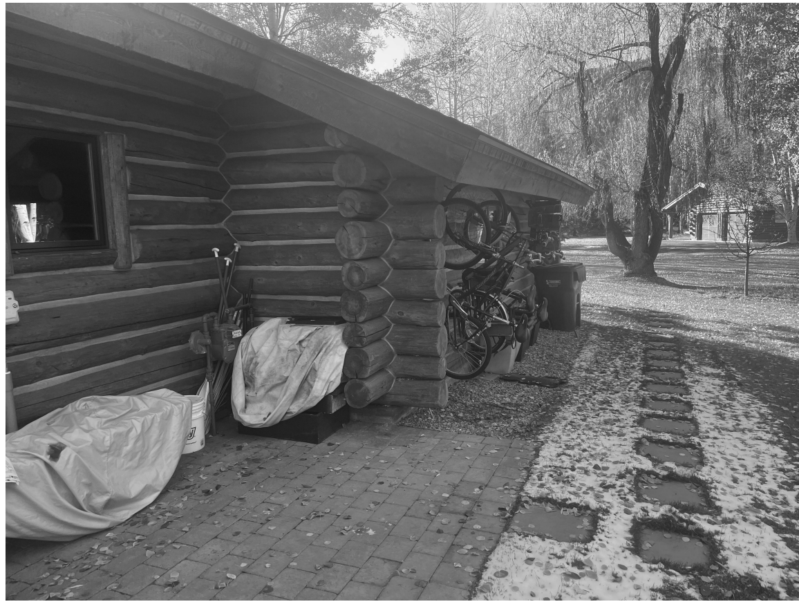
PHOTO #4 - GAS METER TO BE MOVED AS REQ. THIS STORAGE AREA TO BE REMOVED.
